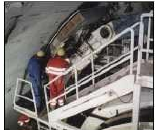
Forming a ring of tubbings
